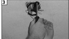
Use metal outlet box suitable for fan support and use only the screws provided with the outlet box (must support 35 lbs). Before attaching fan to outlet box, ensure the outlet box is securely fastened by at least two points to a structural ceiling member ( a loose box will cause the fan to wobble). **Use only the screws provided with the outlet box.**
